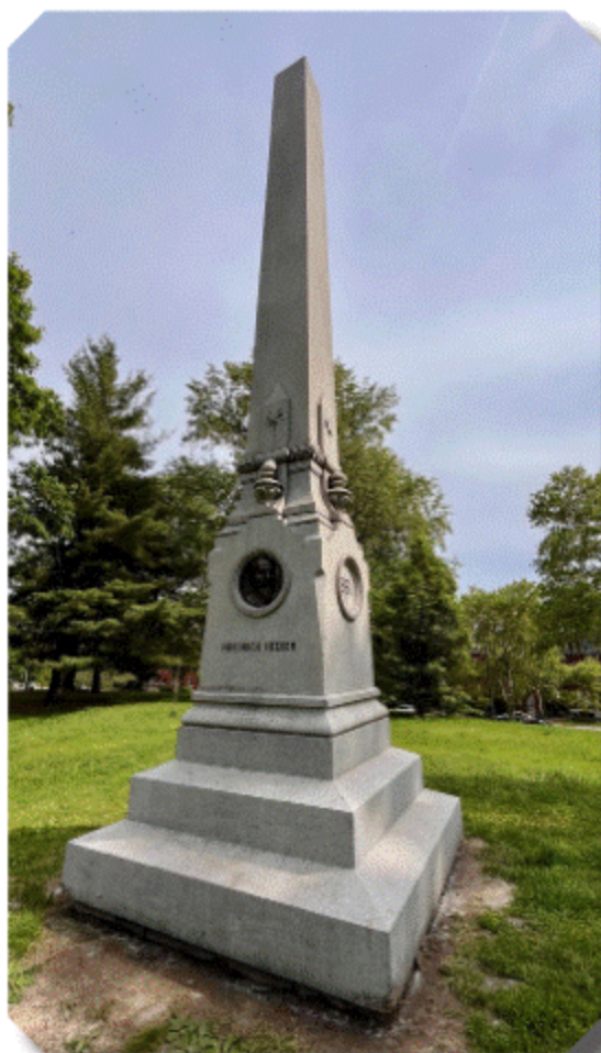
Restoration of the Hecker Monument
