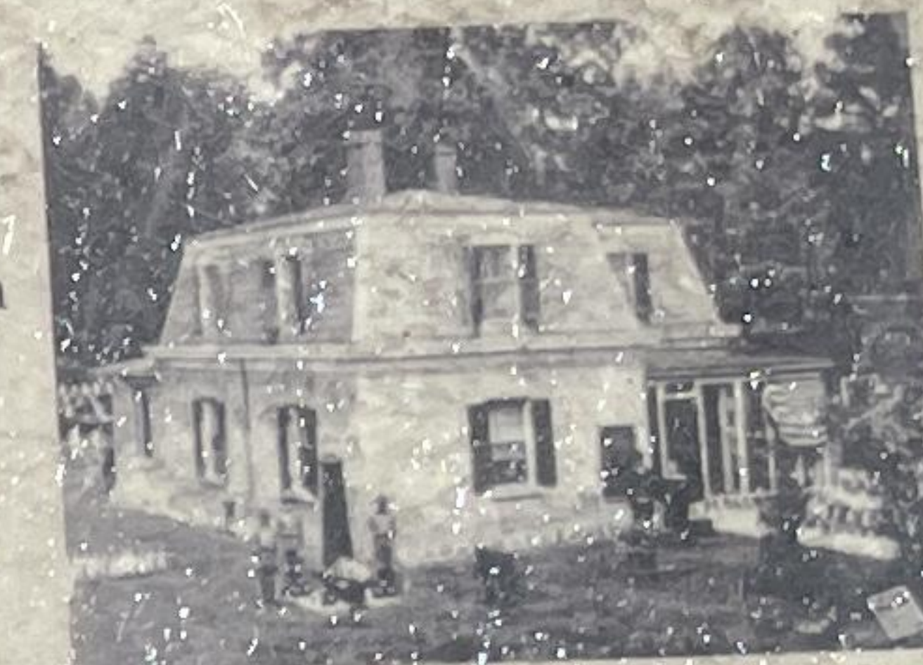
Lodge at City Point, Va., pre-1928. The first floor contained a cemetery office, and living room and kitchen for the superintendent's family; three bedrooms were upstairs.
