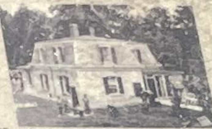
Lodge at City Point, Va., 1862. The first lodge provided a cemetery office and living space and kitchen for the superintendent's family and his own staff.
