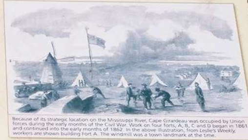
Because of its strategic location on the Mississippi River, Cape Girardeau was occupied by Lincoln's forces during the early months of the Civil War. Work on four forts, A, B, C, and D began in 1861 and continued into the early months of 1862. In the above illustration, from Leslie's Weekly, workers are shown building Fort A. The windmill is a town landmark at the time.
