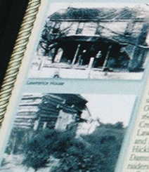
The home of the late James Lawrence was the principal target of John Brown's raid. The log building is said to be a slave cabin on the Lawrence farm. The farmstead was situated west of this location.
