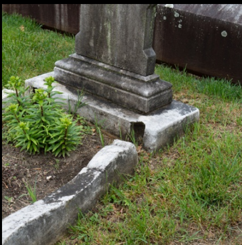
Stabilize ground and reset stones. Repair and reset cradle headstones.
