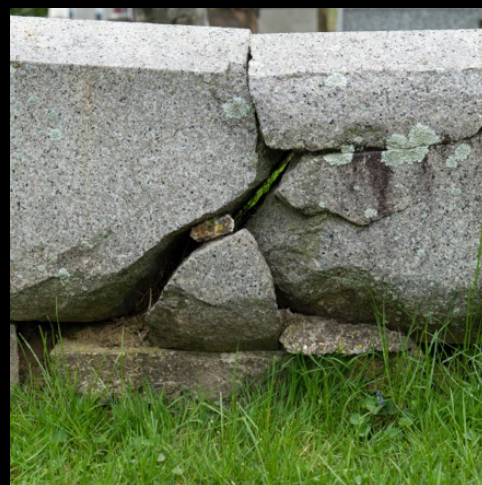
Repair, replace, and reset granite coping.
