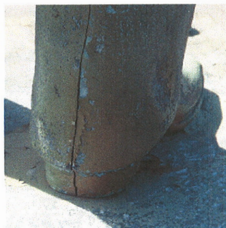
Crack in leg
