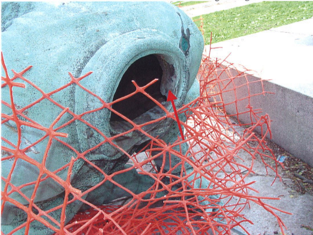
Shown: Soldiers and Sailors Monument, Boston, MA. Vandalized “The Soldier” statue. Note: Corrosion inside collar. Bolt holding head on was snapped. Statue head was recovered. Corrosion and staining damage.
