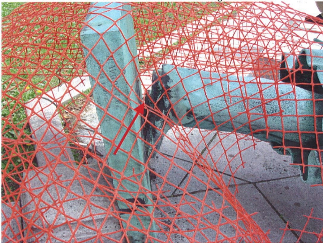
Shown: Soldiers and Sailors Monument, Boston, MA. Vandalized “The Soldier” statue. Note: Statue feet pulled away from base. Base bent and stressed at toe of shoes. Some corrosion damage.
