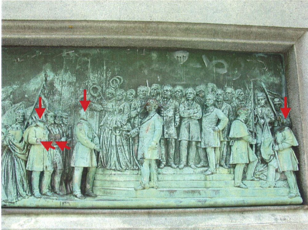
Shown: Soldiers and Sailors Monument, Boston, MA. "Departure for the War" bronze relief. Note: Numerous heads, arms, legs, rifles are missing. Some corrosion and graffiti damage.
