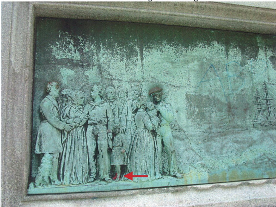
Shown: Soldiers and Sailors Monument, Boston, MA. "The Navy" bronze relief. Note: Corrosion and graffiti damage.
