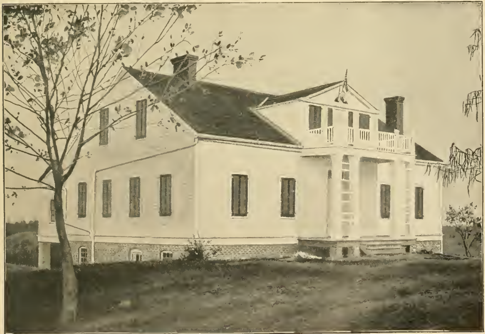
Front and west end view after restoration
