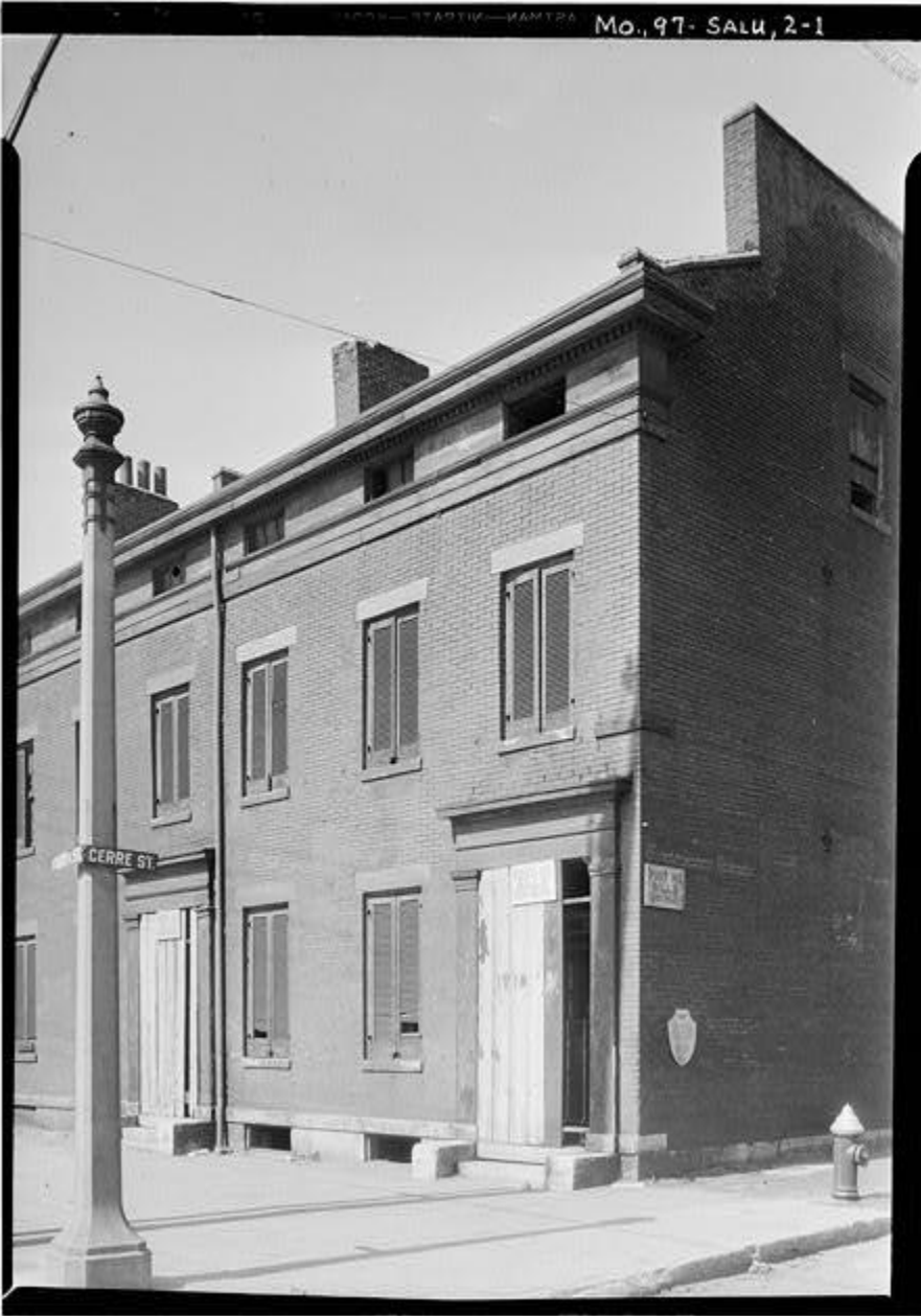
Original building, Alexander Piaget, Photographer, April 10, 1934 VIEW FROM NORTHEAST
