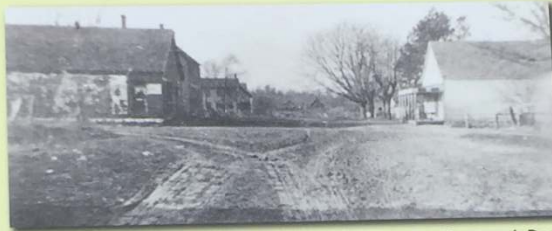
Looking west on the corner of Thome and Spring Street at Spurgeon's Dry Goods Store, which may have been used as a battle hospital. Courtesy Bertha Doud Parke
