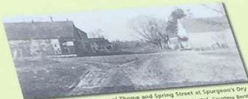
Locking went on the corner of Thome and Spring Street at Spurgeon's Dry Goods Store, which may have been used as a battle hospital. Courtesy Bertha Doud Parks
