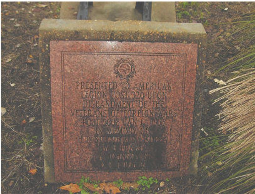
Granite Plaque set in Concrete. The concrete is 4 inches at the top and is 12 inches at the base. It's shape is such that the front slopes back in order to make it easier to read. The granite is stained towards the bottom with the stain coming from the cannon. Text of the plaque is on the form.
