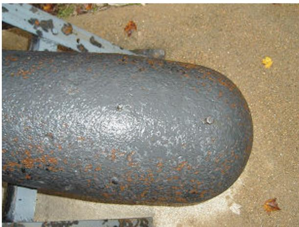
← The breech of the cannon shows rust coming through the paint. It has a metal pin and a bolt in it. The pin looks like an aiming device. The barrel at the back is 12 inches wide. The Knob and the neck was either broken off or cut off
