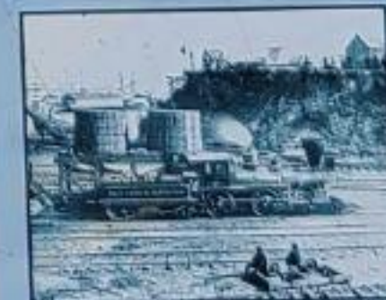
The Union Corps of Engineers laid tracks and built bridges for the military trains. Courtesy Library of Congress
