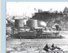
The Union Corps of Engineers laid tracks and built bridges for the military trains.
