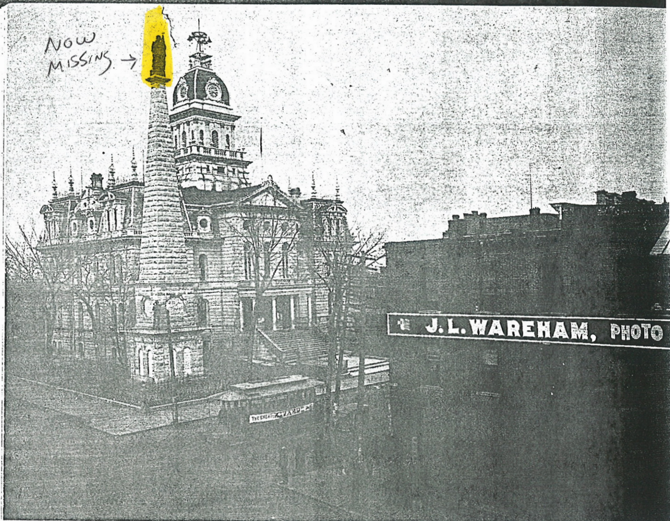
The Stephenson County court house and soldiers' monument about 1896 showing full detail of ironwork and trim as well large clock tower.
