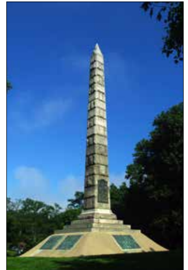
Figure 154. North Alton Confederate Monument was completed in 1910; its original earthen base was covered in concrete, probably by WPA labor repairing the foundation in the 1930s.
