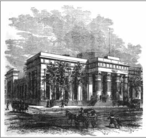
Figure 96. The Tombs, ca. 1870; the building was razed in 1902. Appletons' Journal, "New York Illustrated. No. 1" Art Supplement, April 24, 1869.
