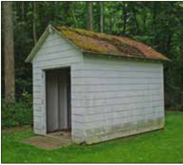
Figure 180. Former utility shed behind the Point Lookout monument.
