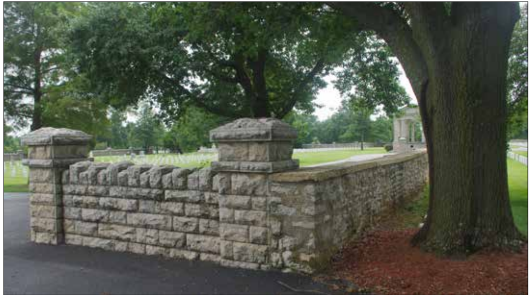
Figure 204. The intersection of the original Springfield National Cemetery wall with its simple coping (right), and more ornate Confederate cemetery wall (left); utilizing the national cemetery wall saved the UCV several thousand dollars.
