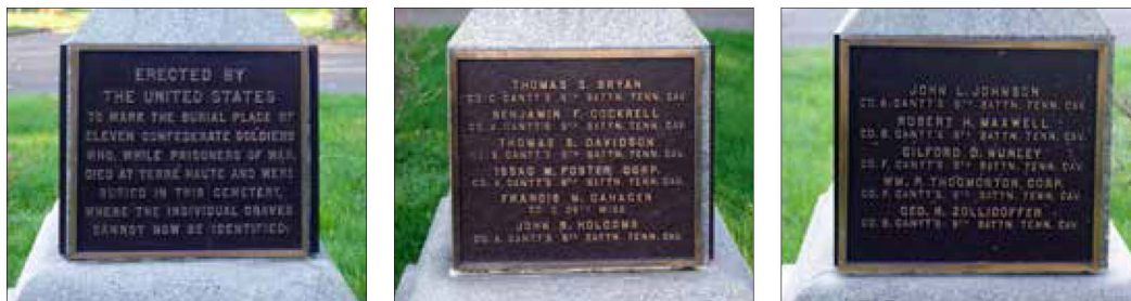
Figure 216. Plaques added to the monument when it was moved in 1951: recognition (leftmost), and two on the east and west faces inscribed with names of the dead.
