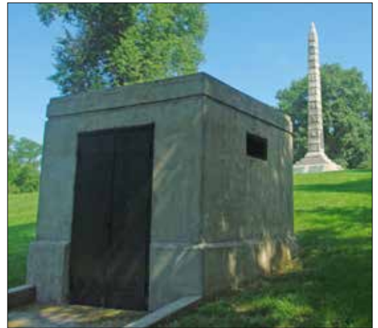
Figure 158. The concrete storage shed at North Alton in 2009.
