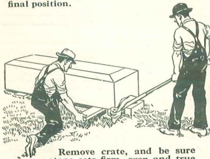
Remove crate, and be sure stone sets firm, even and true on foundation.
