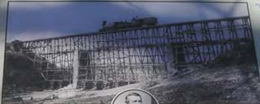
The Potomac Creek Bridge (under construction), ca. February 1862, looking across the creek from a viewpoint located just down the slope in front of you.
