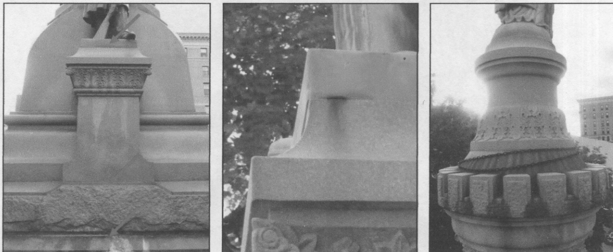
Figures 21-23. Examples of copper staining (left), mild and significant rust staining (center and right, respectively) on the monument.
