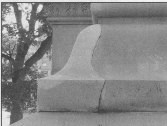
Figure 10. Point-loading has caused one corner of the cyma level to separate at a fracture line.
