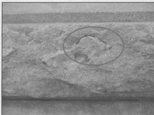
Figure 9. Minor incipient spalls on the face of the base stones are due to the original technique used to create the pitch-faced finish of the stone.
