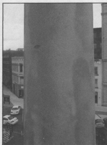
Figures 13-15. The stone exhibits some unevenness of color due to variations in weathering (left and center), leaving some minerals more exposed (detail, right).
