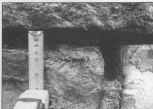
Figures 17 and 18. Example of a typical lead strip caulk dislodged from its joint (left) and one of the many wide, open joints of the foundation (right).
