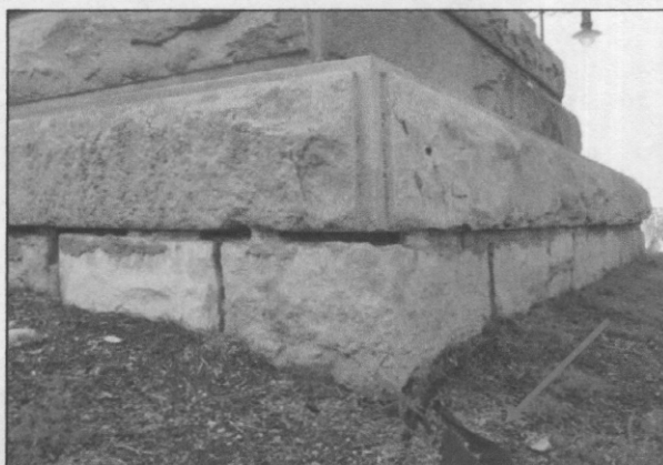
Figure 16. General condition of the foundation (lower course). Also note the emergence of the landscape fabric.
