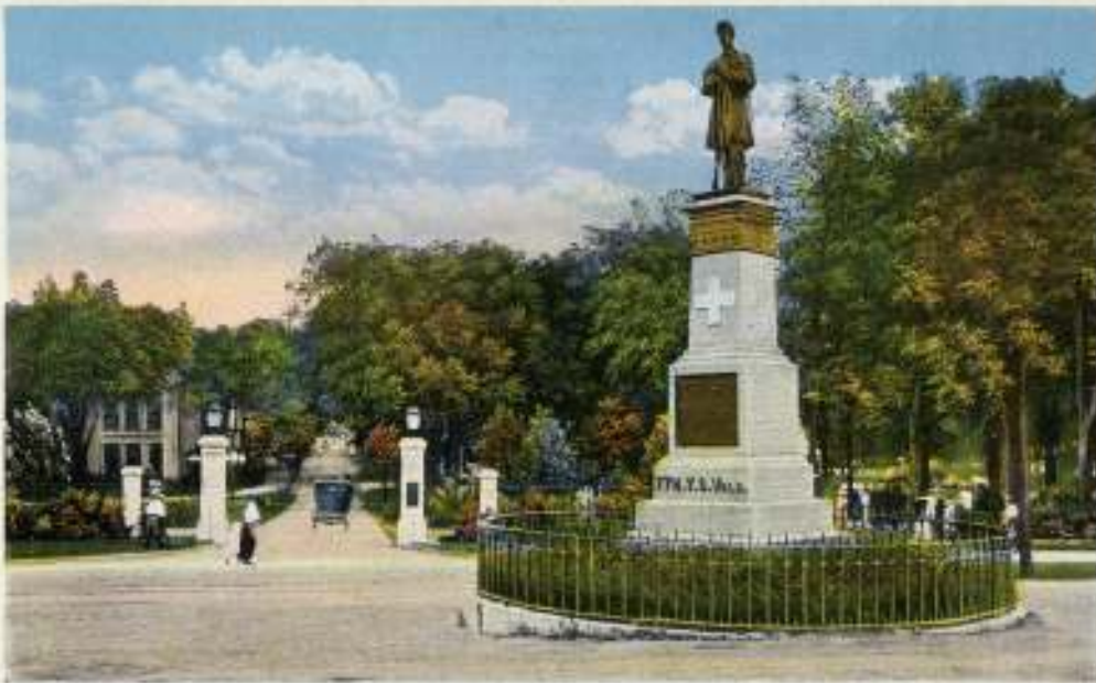
SOLDIERS MONUMENT AND ENTRANCE TO CITY PARK, SARATOGA SPRINGS, N. Y.
