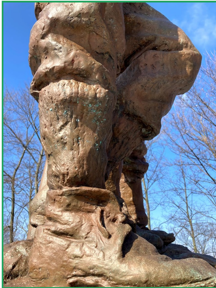
Oxidation/corrosion on sock.
