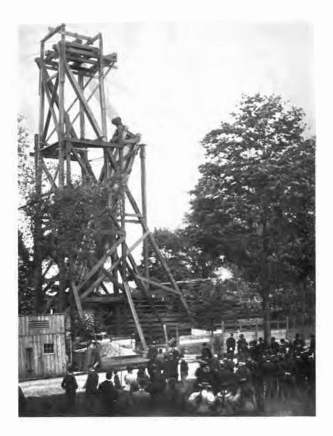
This trial developed a weakness in the front brace timbers, which was remedied by adding more guys to the back. When the final lift was made, everything worked smoothly, and in ten minutes the shaft was erect and resting on the stone post.
