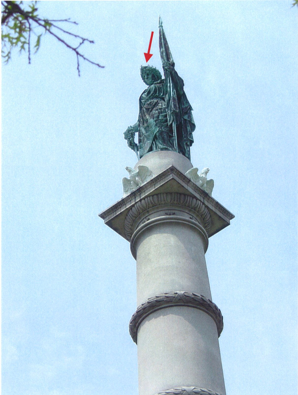
Shown: Soldiers and Sailors Monument, Boston, MA. "Genius of America" statue atop monument column. Note: Star missing in crown on statue. Some corrosion damage.
