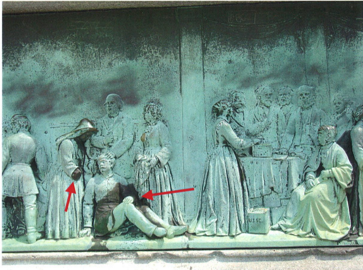
Shown: Soldiers and Sailors Monument, Boston, MA. "The Sanitary Commission" bronze relief. Note: Arm missing. Some corrosion damage and staining.
