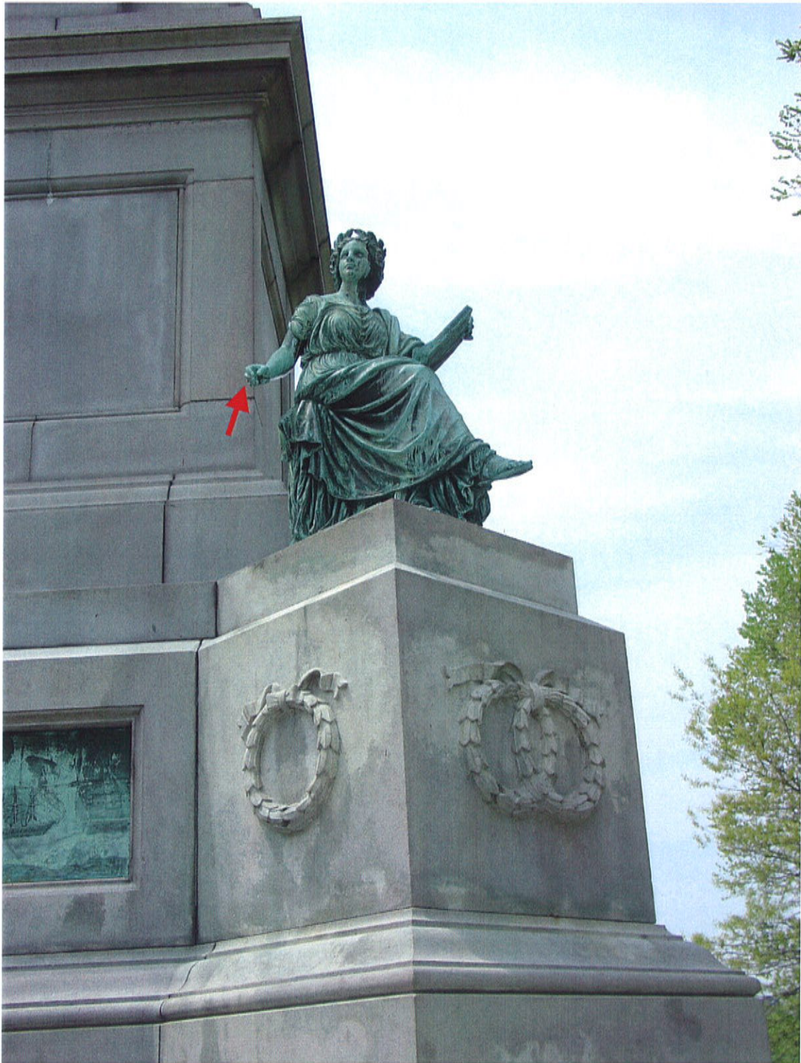
Shown: Soldiers and Sailors Monument, Boston, MA. Note: "History" statue missing stylus from right hand. Some corrosion and staining damage.
