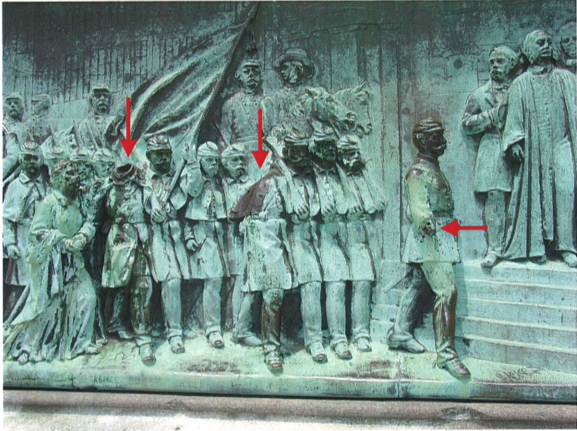
Shown: Soldiers and Sailors Monument, Boston, MA. "Return from the War" bronze relief. Note: Heads, arms and part of a torso missing. Some corrosion damage.
