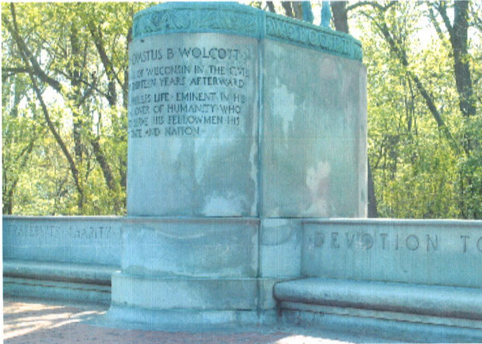
Fig. 7. Detail of the inscription. The stone is unevenly stained. None of the original bronze letters are found at the moment on the monument. Only indentations in the stone are present, but the inscription is readable due to precise carving in the stone.
