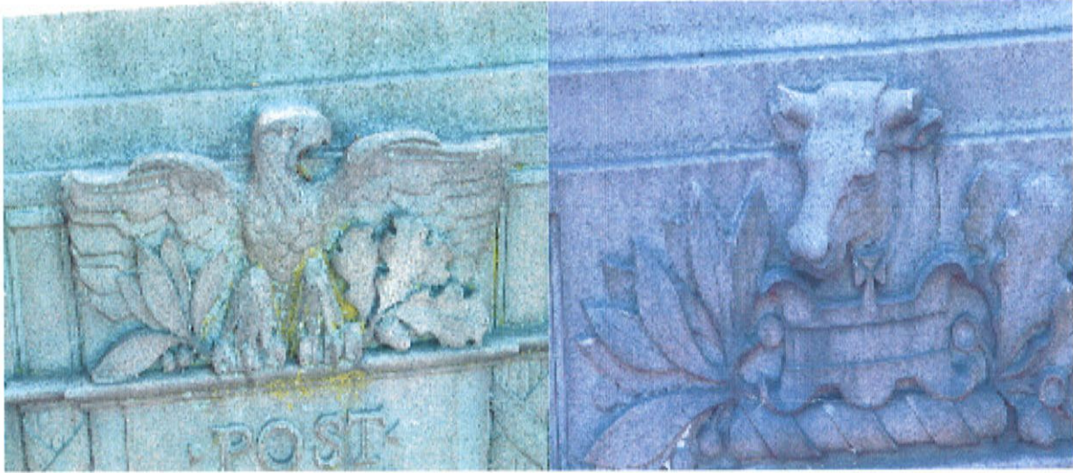
Fig. 13. Detail of the carved stone from the proper left and right side of the bench. Please note discoloration of the stone, and missing horns of the bull. The surface of the stone is covered with biota.
