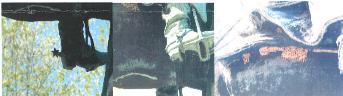
Fig 5. Detail of the proper right leg of Wolcott - showing streaking, four mud wasp nests, and leaching of what appears to be a core material from
