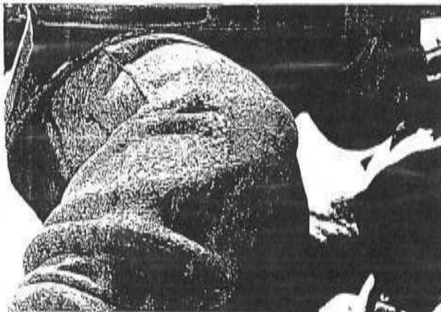
Fig. 7. Proper right soldier - proper right knee. Note, a gray core material is leaching from the inside of the sculpture.
