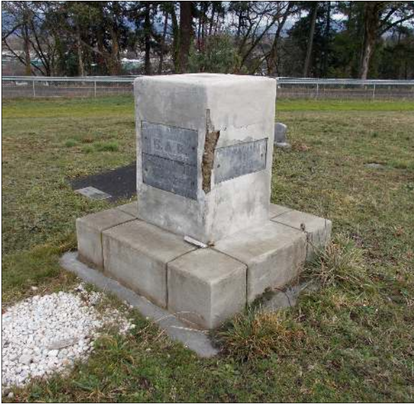
Current state of the monument - January 2021.
