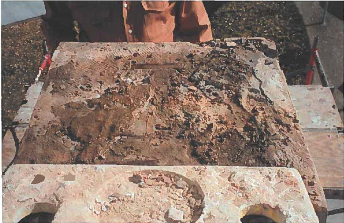
4. During – Mortar Bed of A1 with Iron
