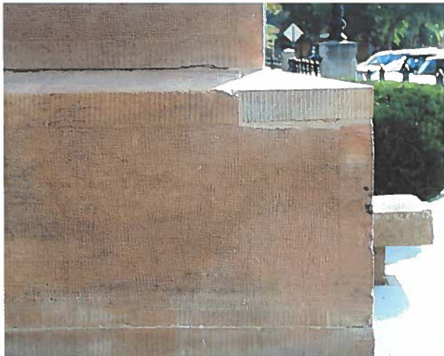
15. After – C1 replaced stone ledge at south corner, west side.
