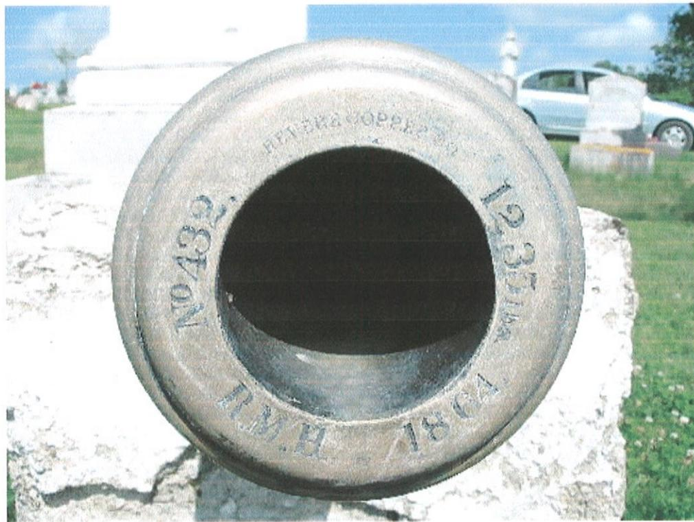
Markings on Muzzle/Left Trunion - #1 – Federal Acceptance #427, Casting #438, Revere Copper Co., 1238 lbs., 1864 (Date of Acceptance), RMH (Person in charge and Acceptance)
