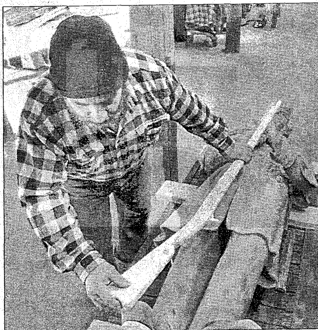
Peter Crockett of Argyle, an artist and pipe welder hired by the Orono Historical Society to refurbish the town's Civil War monument, demonstrates where the soldier's new gun will be placed.
