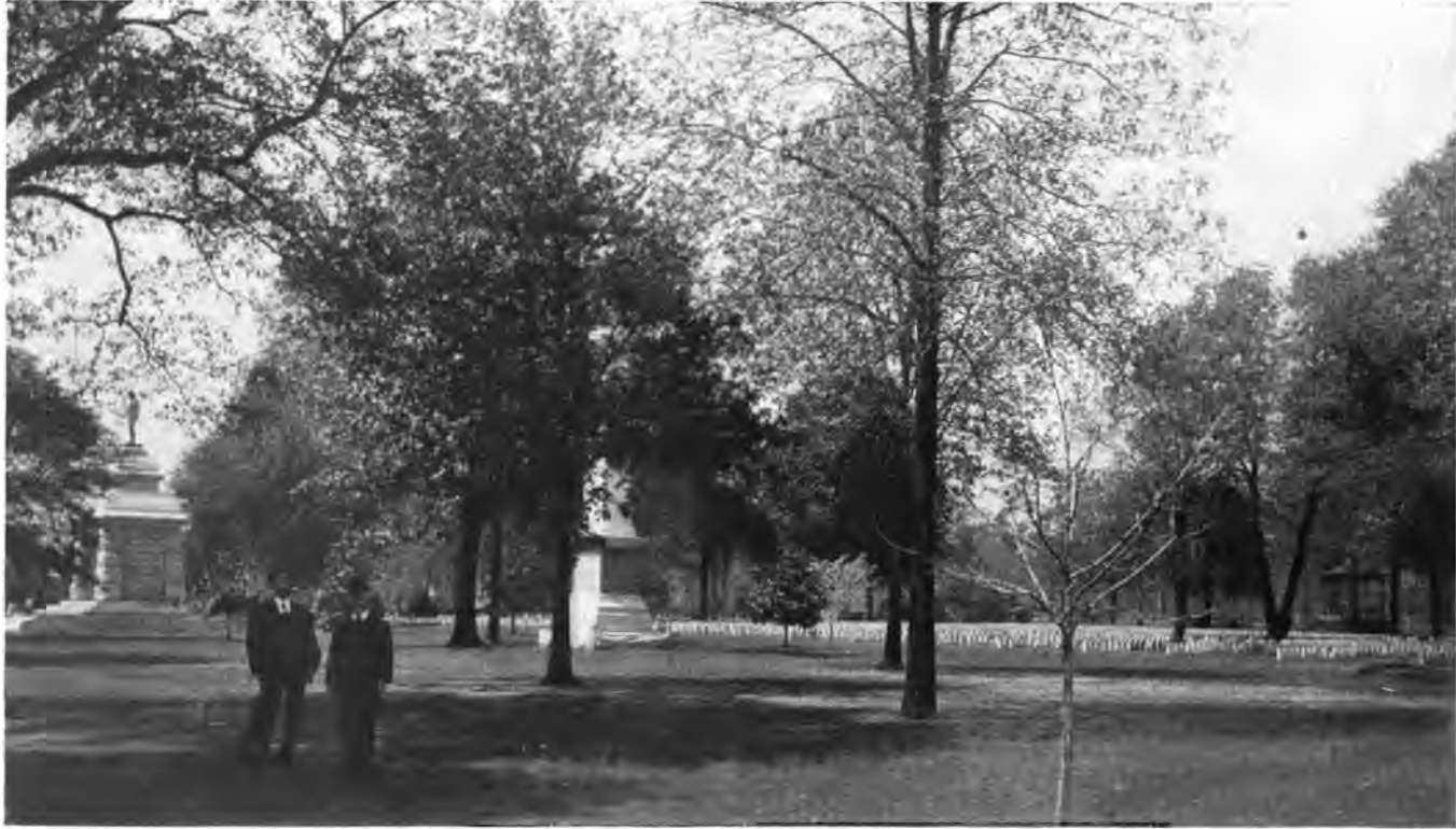
NORTHWEST SECTION, SHOWING PENNSYLVANIA AND MAINE MONUMENTS
