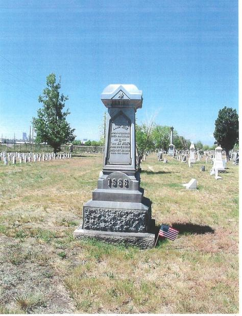
Because it is zinc, the metal of the memorial appears chemically sound; it has not corroded. Lettering remains clearly legible. The sculpture has produced a self-protective patina.
