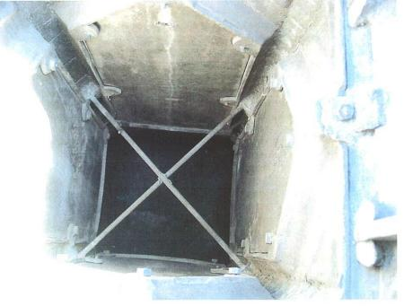
The interior view illustrates bolts securing sections across cast joints. The "X" is a pair of tie rods placed inside the tall center section to aid in keeping the Memorial square.
